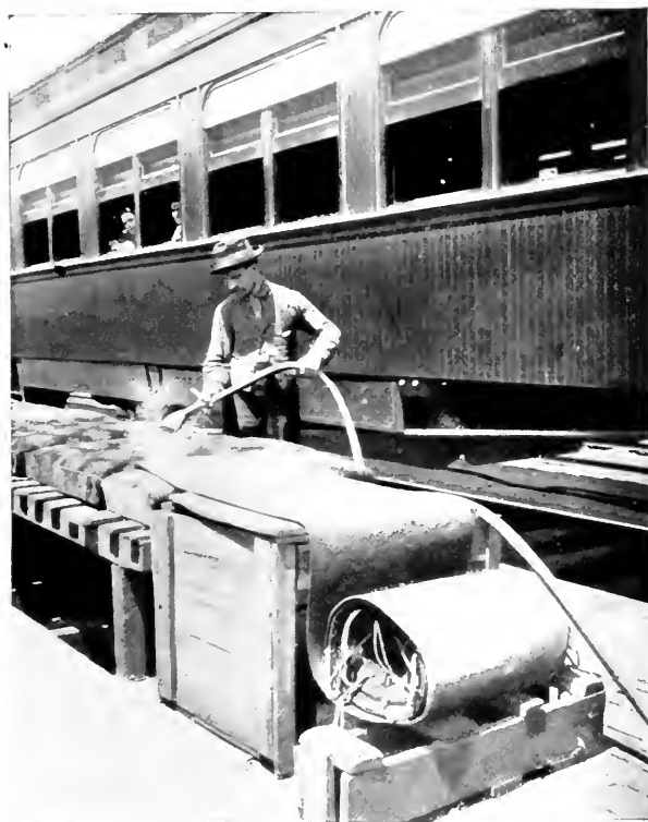
FIG. 7. CLEANING CAR CUSHIONS WITH AIR.
